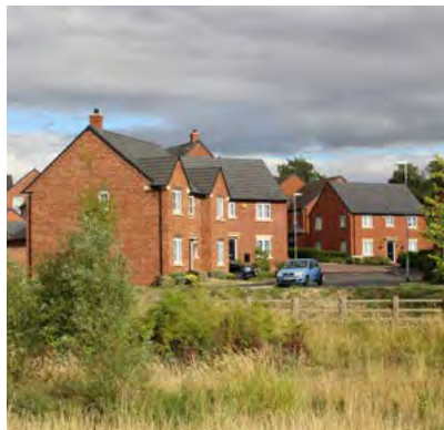
Black front doors and porches, simple cast stone lintels
