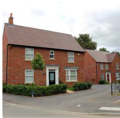
Private driveways serve a handful of homes fronting green spaces
