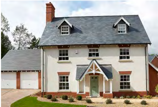
Examples of high quality housing delivered by Barwood
