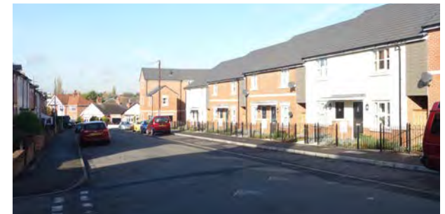
Modern, more recent housing development to the south of Sileby on Cemetery Road using a mixture of local brick, banding details and white render
