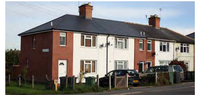
Lower density, 1950s suburban terraces on Ratcliffe Road, usually in runs of four and featuring part brickwork and part rendered façades in this example
