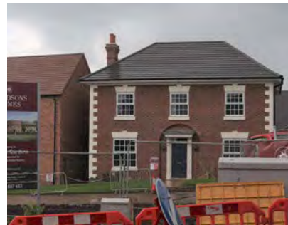
Gateway development under construction
